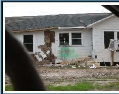
Asbestos Home After Hurricane
